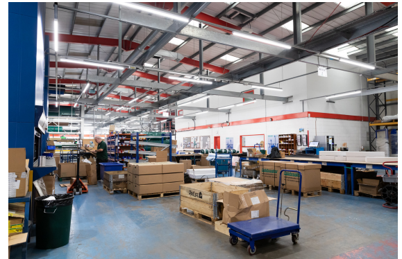
Galebreaker assembly area, showing the lighting installed with help from BEEP support
